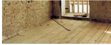
View of a floor after removing the substrate and flooring existing before it was strengthened.
