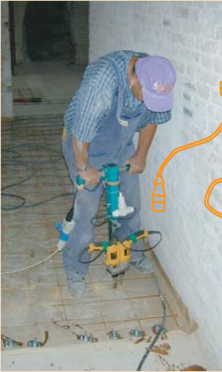
Holes drilled in boarding and beam with a double drill. This tool is available for hire.
