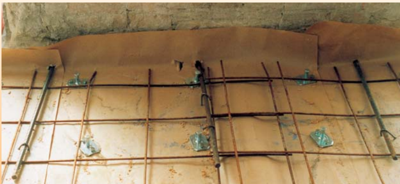
Holes drilled in boarding and beam with a double drill. This tool is available for hire.
